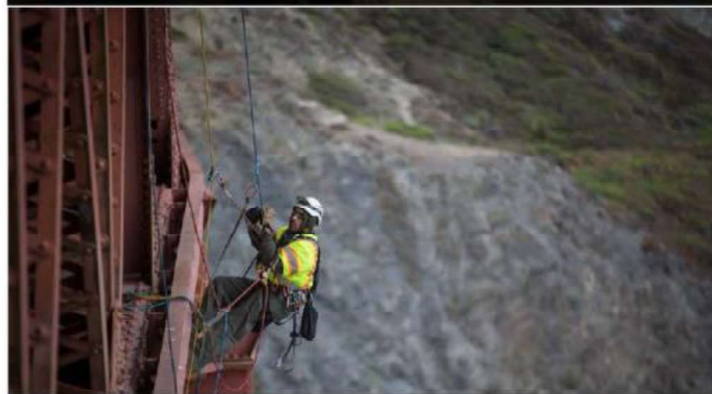
Golden Gate Bridge, Fracture Critical Inspection Services
