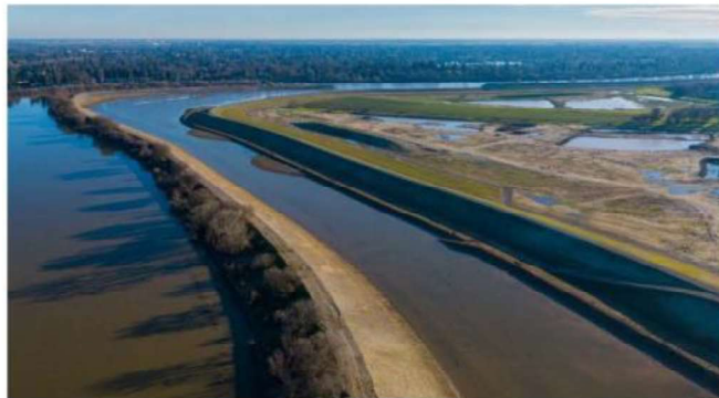
Southport Levee Improvement Project
