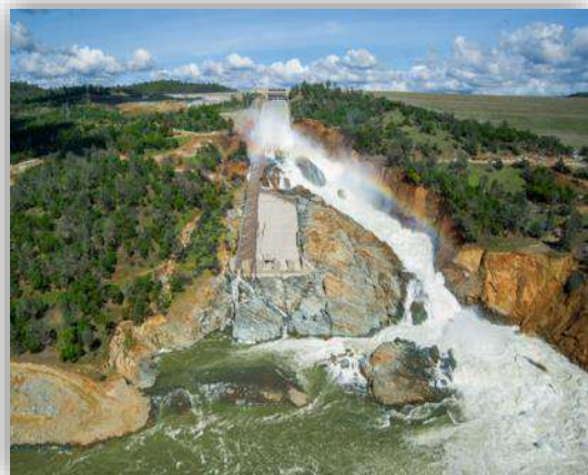
CFD Model Results for the Damaged Spillway Condition (Oroville, CA)
