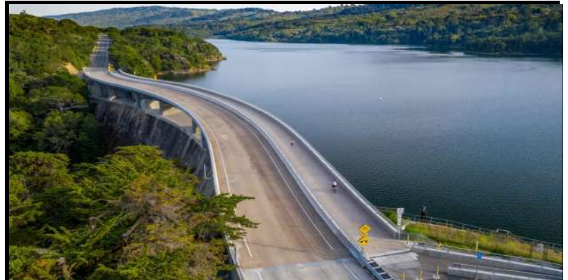
Crystal Springs Dam Bridge
