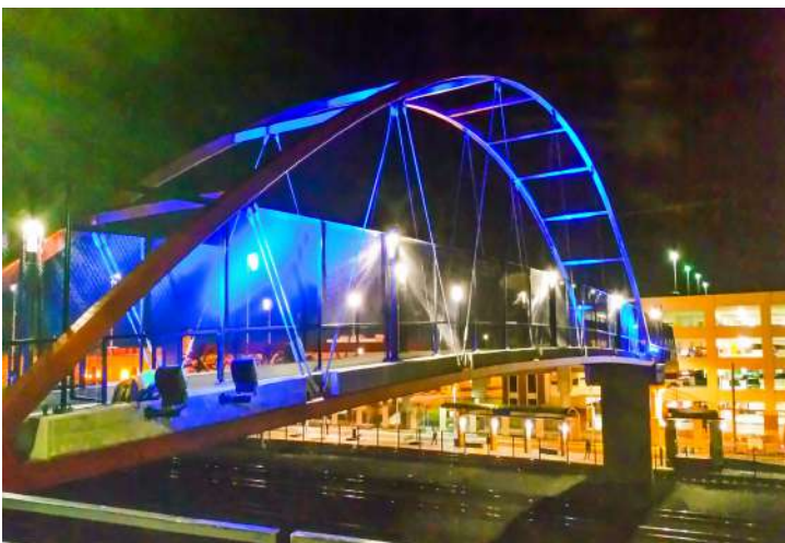
City College Light Rail Station Pedestrian/Bicycle Crossing. Sacramento, CA
