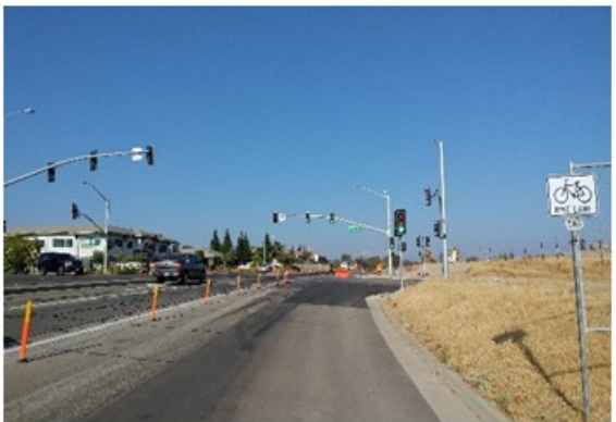
Turn Lane Addition – Sierra College Blvd, Rocklin, CA
