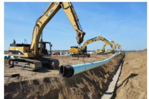
Stormwater Force Main Pipe
