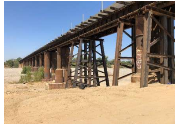
UPRR 2,568-ft-long bridge over the Yuba River.
