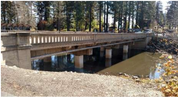
Fanny Bridge Retrofit, Tahoe City, CA
