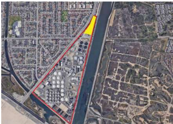
GWRS site at OCSD's Plant 2 site in Newport Beach, CA
