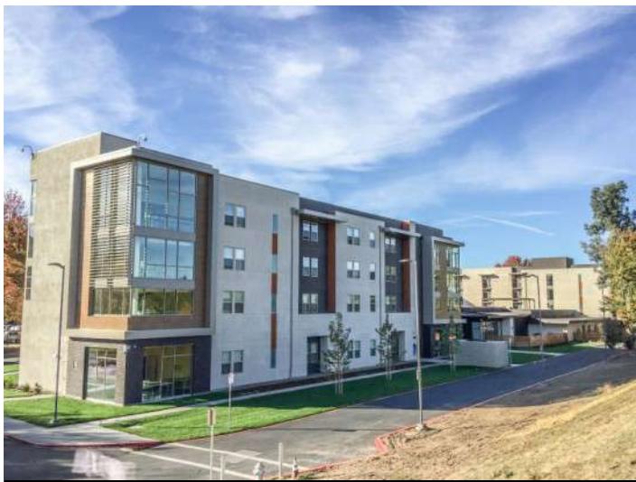
Sacramento State Student Housing photo: BKF was part of the design team for a new 4-story student housing building for Sacramento State University along the American River in Sacramento.
