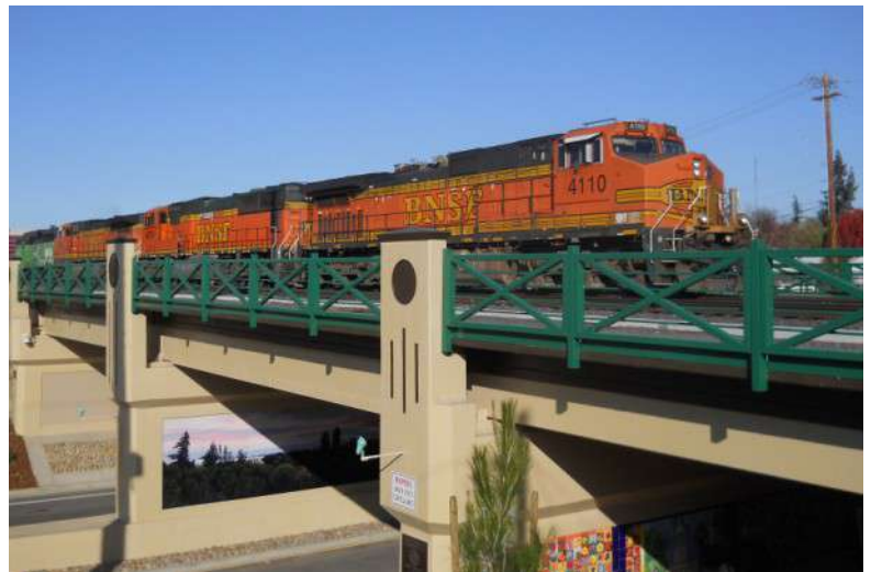
G Street Grade Sep photo: BKF was the civil engineer for the G Street grade separation project that created an underpass for G Street beneath the BNSF railroad in Merced.
