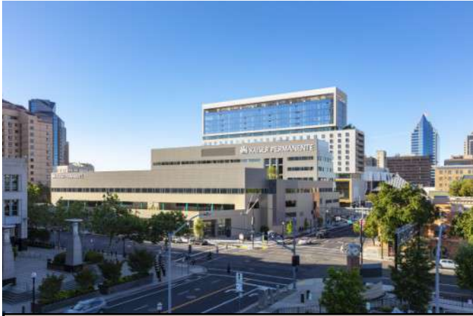
Kaiser Capital Gateway MOB photo: BKF provided civil design for the conversion of existing office building at J Street in Sacramento, CA to a full service medical office building.
