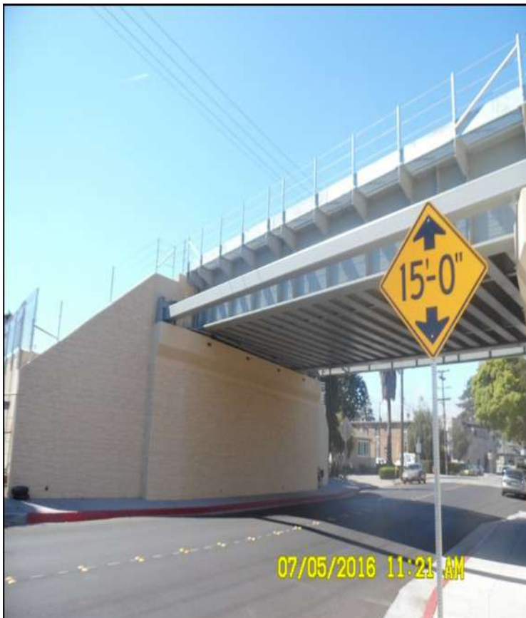
Completed Polar Avenue Caltrain Bridge
