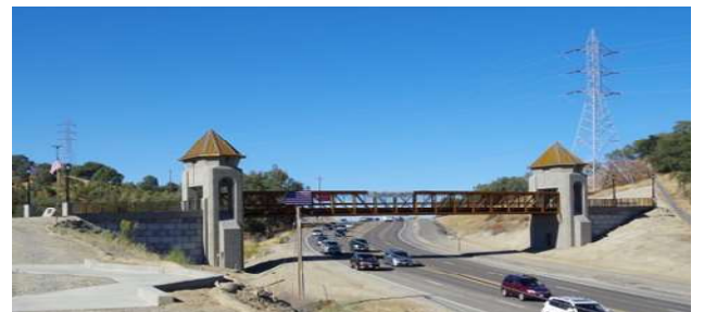
Johnny Cash Pedestrian Bridge
