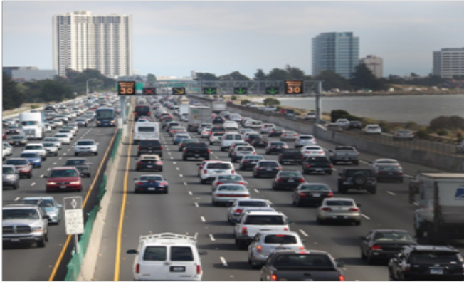
I-80 Integrated Corridor Management Project
