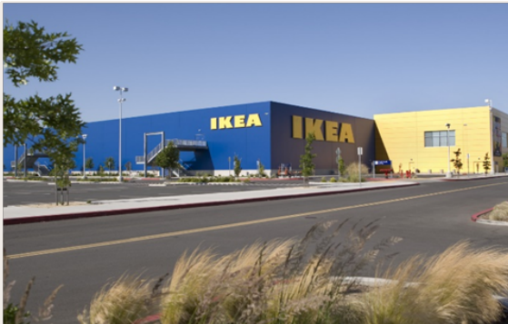
West Sacramento IKEA Site Development
