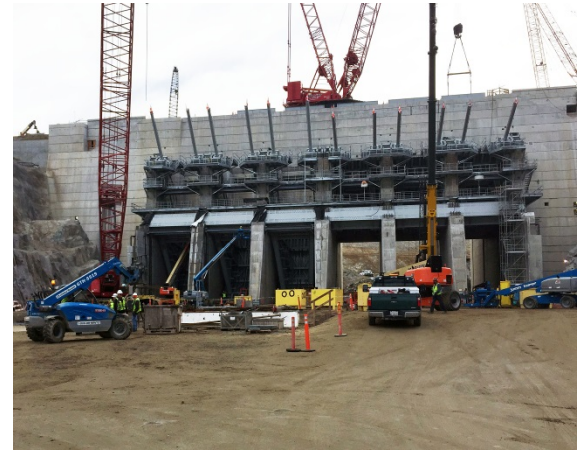
Folsom Dam Auxiliary Spillway Folsom CA
