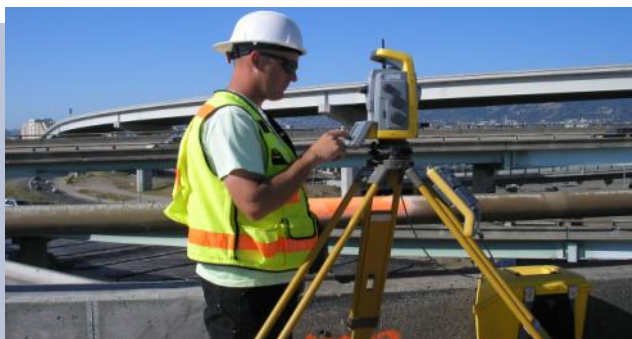
I-580 Bridge Collapse 018
