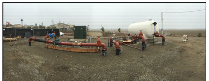
"The Cannery" Agricultural Well The New Home Company, Davis, CA
