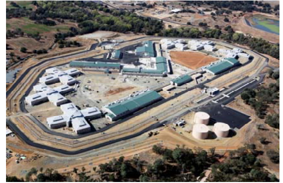
Mule Creek State Prison Expansion Design-Build Project, Ione, California
