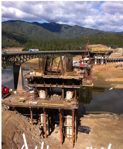
Antlers Bridge Project, Lakehead, CA
