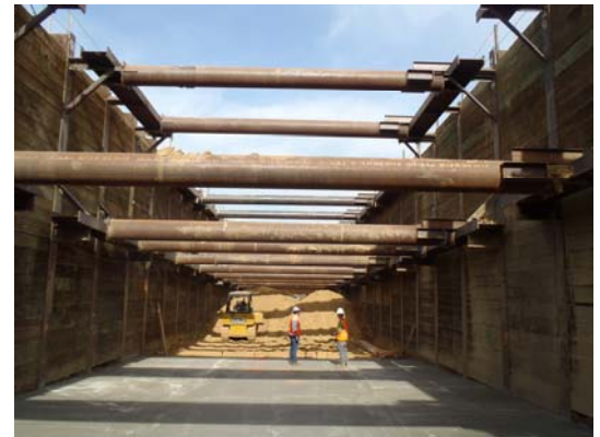
Crenshaw 1, Southern California Temporary excavation support systems for subterranean rail station.
