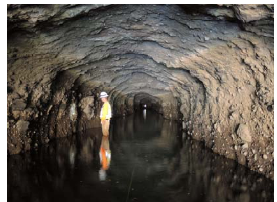
Northern California Tunnel condition assessment
