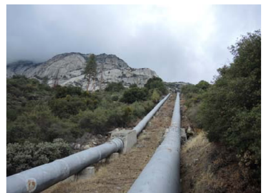
Northern California Geohazards assessment of hillside penstocks.
